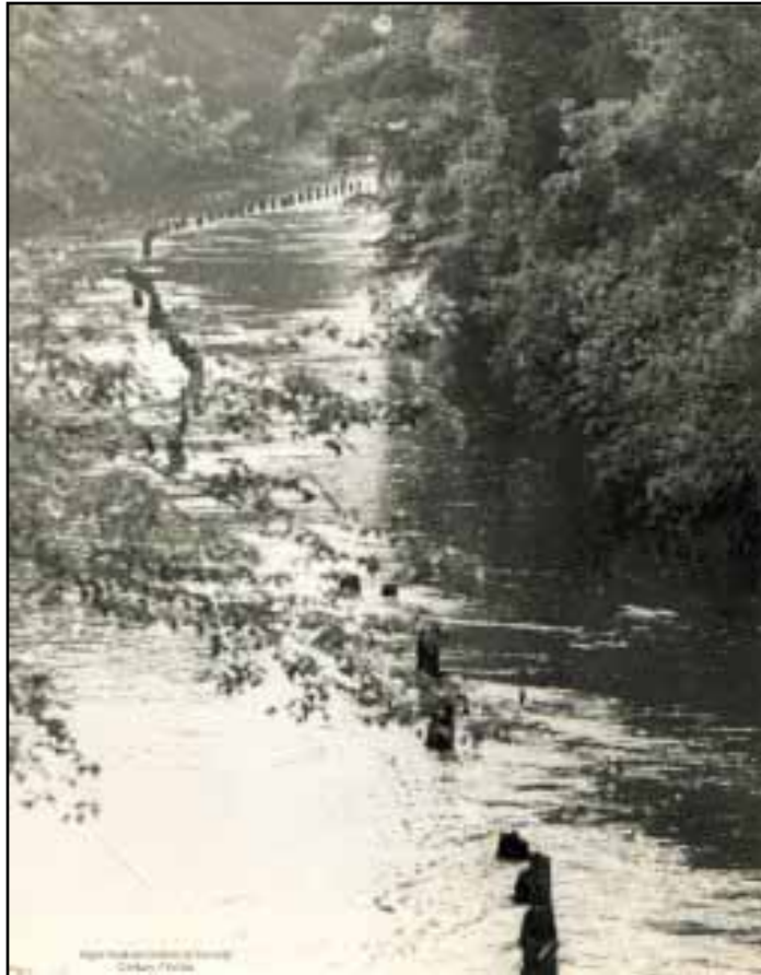
These pilings may be seen on the west side of the twin bridges (where U.S. 31 crosses Little Escambia Creek
